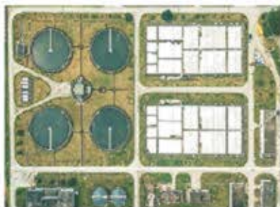
Sewage Treatment Industry
