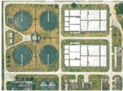
Sewage Treatment Industry
